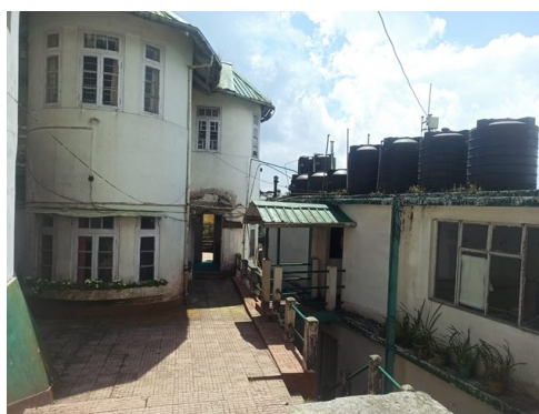
Courtyard & heritage wing — colonial architecture
